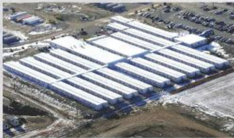
Many workers in the Williston, N.D., area call hastily built crew camps their homes.
